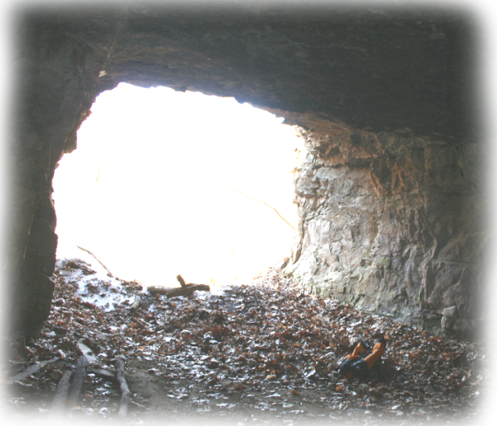
Above: An Illinois mine entrance prior to gating.
